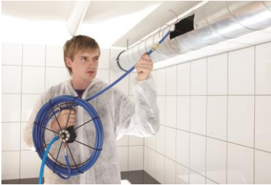
Fig. 22: Application example: Cleaning ventilation ducts
