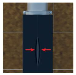
While glueing sheets to the pipe, when attaching the two edges, press them together firmly with your fingers, starting at the far ends, then the centre and lastly along the intermediate points to avoid an irregular joint.
