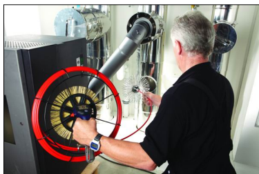
Fig. 20: Cleaning a stainless steel chimney
