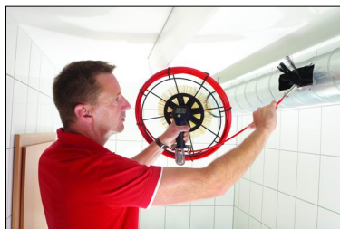
Fig. 21: Cleaning a ventilation duct
